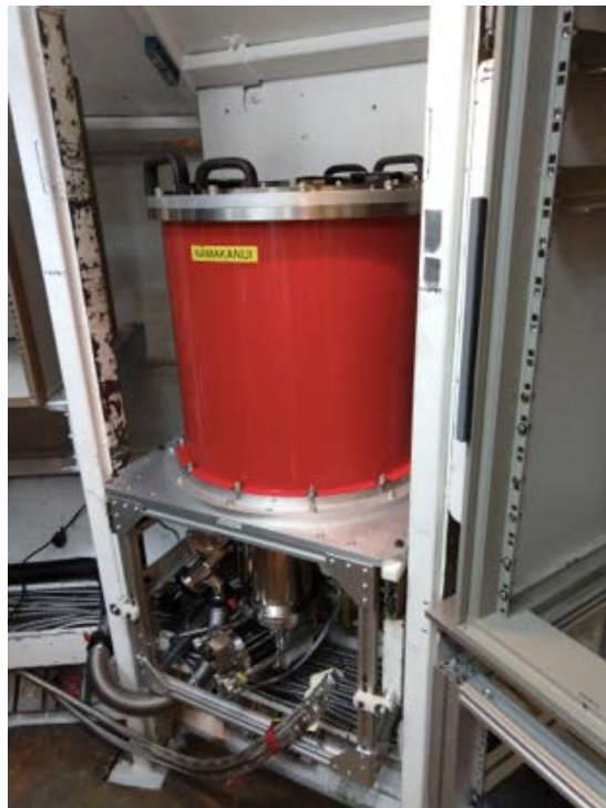
Namakanui (GLT spare): Commissioning
